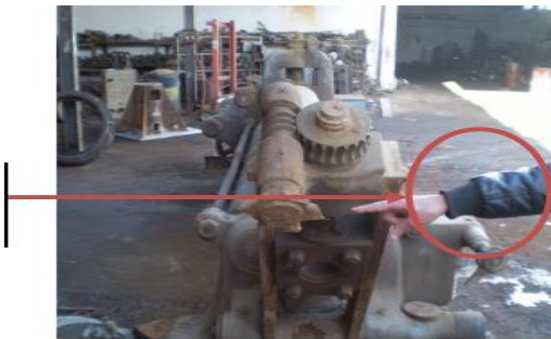
Figure 2: Issue 2 - Flywheel Damage Due to Pulley Malfunction
