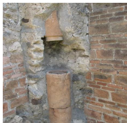
Figure 2 Vertical pipes in Pompeii's walls may once have lead to upstairs toilets [2]
